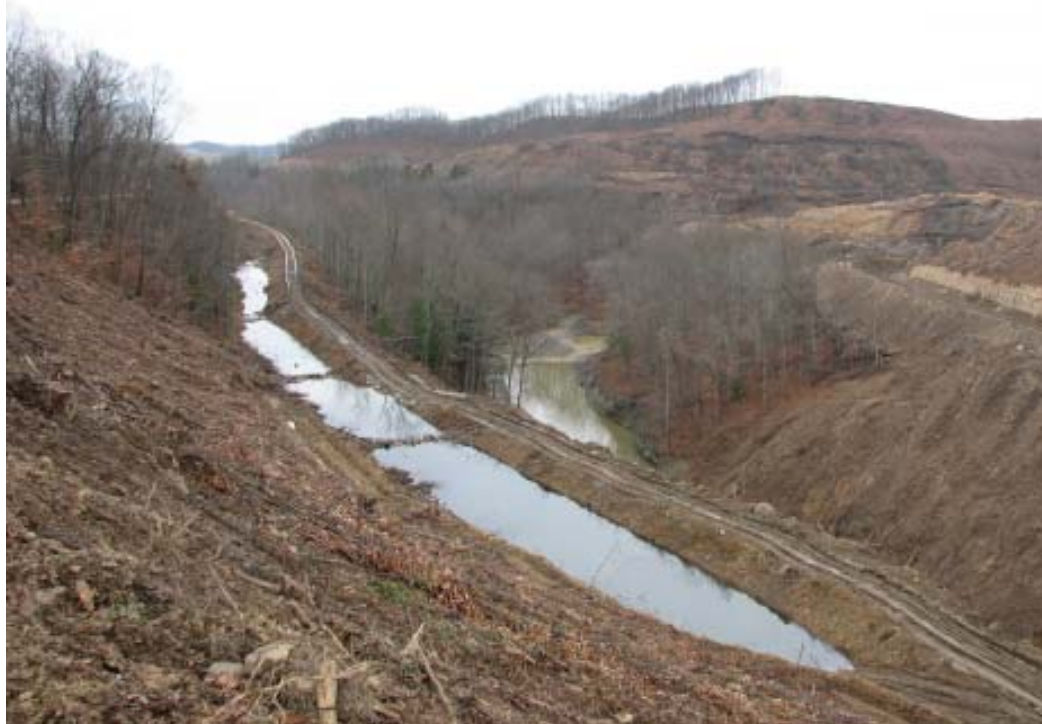
Birds-eye view of drainage ditches, construction road and sediment pond further below - photo by Viv Stockman standing next to our car on county road passing through the operation
