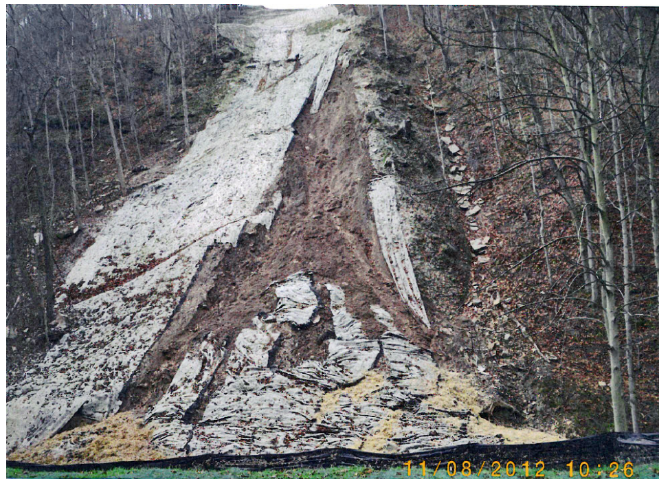
Failure of slope stabilization resulting in stream impact on Dominion's G-150 pipeline in West Virginia. (WVDEP photo)
