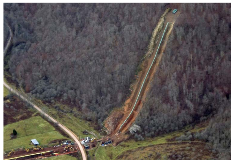
ATLANTIC COAST PIPELINE CONSTRUCTION IN POCAHONTAS COUNTY. WATER BARS ARE NOT INSTALLED AS REQUIRED FOR STEEP SLOPE
