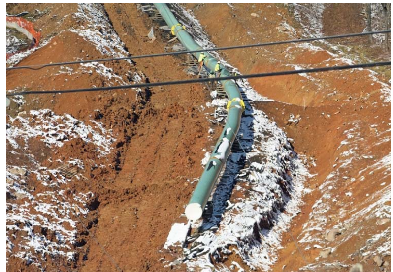
ATLANTIC COAST PIPELINE CONSTRUCTION IN POCAHONTAS COUNTY. WATER BARS ARE NOT INSTALLED AS REQUIRED FOR STEEP SLOPE CONSTRUCTION.
