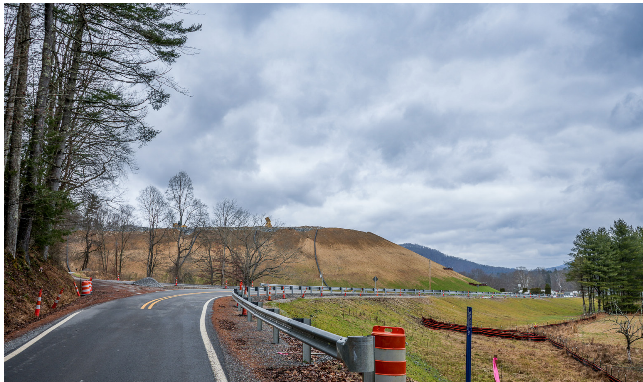
Corridor H construction in Holly Meadows, December 2022.
