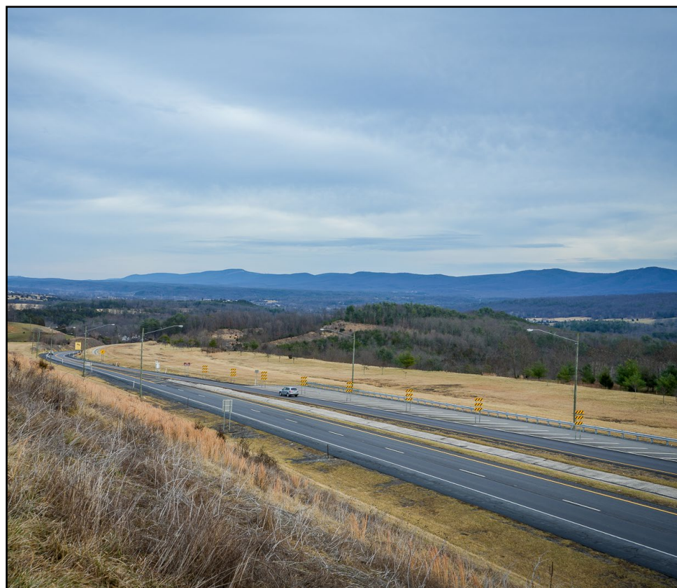
Corridor H segment in Wardensville, WV. (Photo by Olivia Miller)
