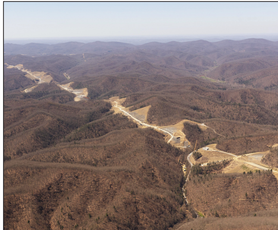
Corridor H section from Kerens to Parsons under construction in 2023. The route has since opened to the public as of June 22, 2026. (Photo by Allegheny-Blue Ridge Alliance)
