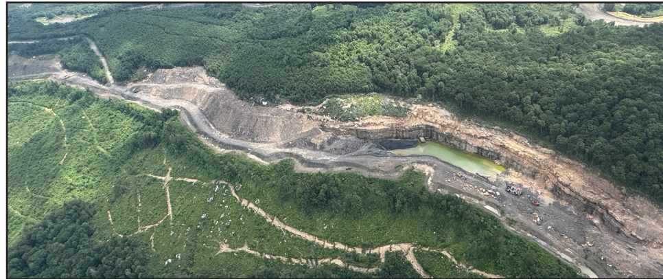
Recent flyover image of Rocky Run Mine and the current damage. (Photo by Allegheny-Blue Ridge Alliance)
